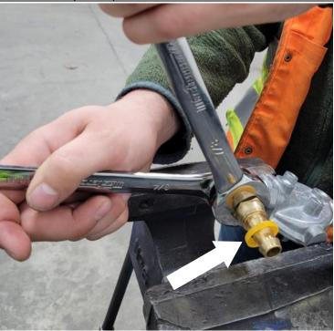
After assembling the fittings on the inlet and outlet ports of the filter head, It is ready to mount on the filter mounting bracket.
